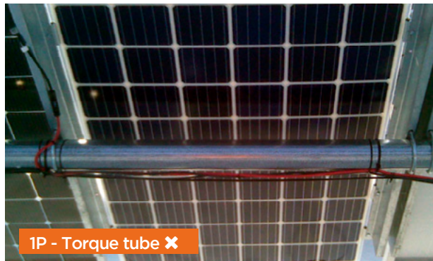
Figure 6- Example of rear shading on 1P and 2P. 6a) 1-in-Portrait 6b) 2-in-Portrait SF7 bifacial Source: BiTEC
