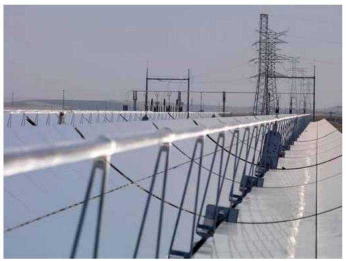
are employed in the solar field in Lebrija. These tubes maximize the absorption of solar radiation concentrated by the parabolic mirror in the receiver placed at the focal line.
