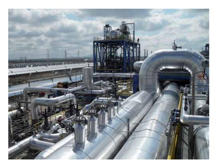
of three units each. The collectors concentrate solar radiation onto solar receivers (UVACs) created by Siemens through which a thermal fluid that absorbs heat circulates.
